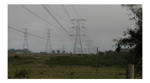
Figure 3.3 : Photograph of conductors strung between transmission towers.
