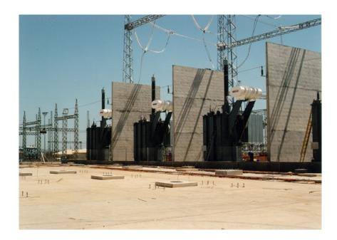
Figure 3.5: Transformers at a Substation.
